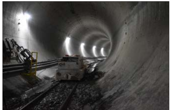
Waterway Protection Tunnel
