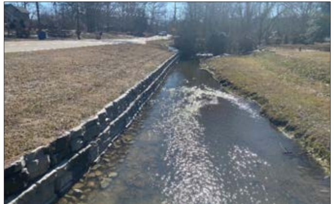
Mount Holly bank stabilization
