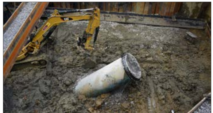
Harrods Creek sewer repairs
