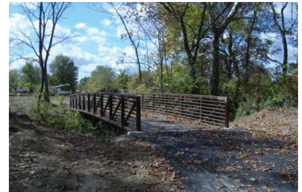
Existing Bridge along Louisville Loop
