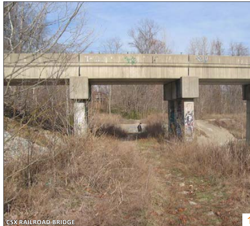
CSX RAILROAD BRIDGE
