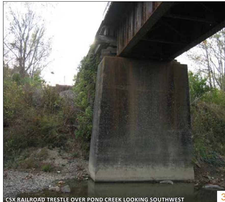
CSX RAILROAD TRESTLE OVER POND CREEK LOOKING SOUTHWEST
