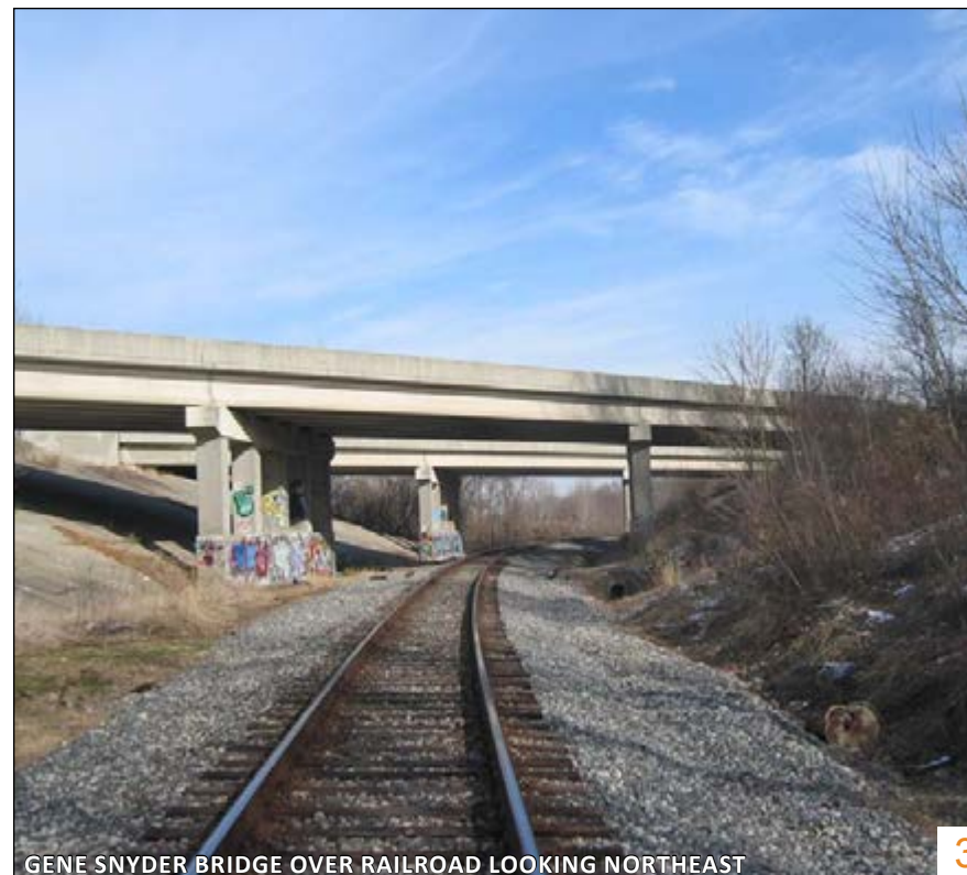
GENE SNYDER BRIDGE OVER RAILROAD LOOKING NORTHEAST
