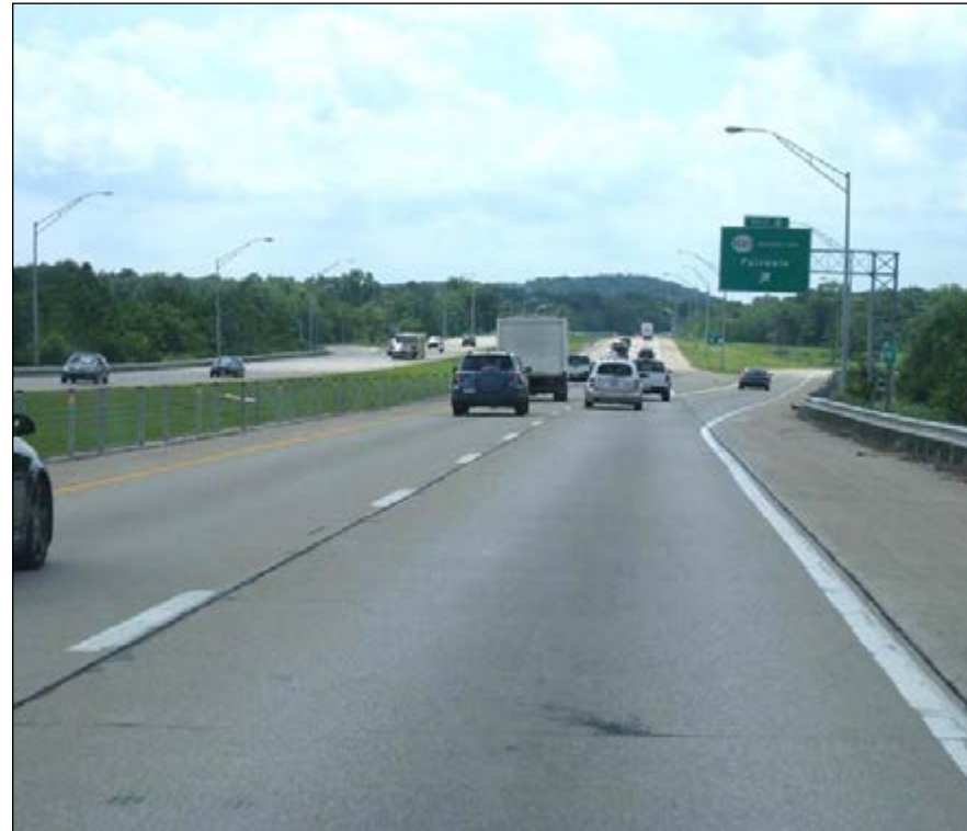
FIGURE 3.19 BARRIER TO PATH CIRCULATION: GENE SNYDER FWY
