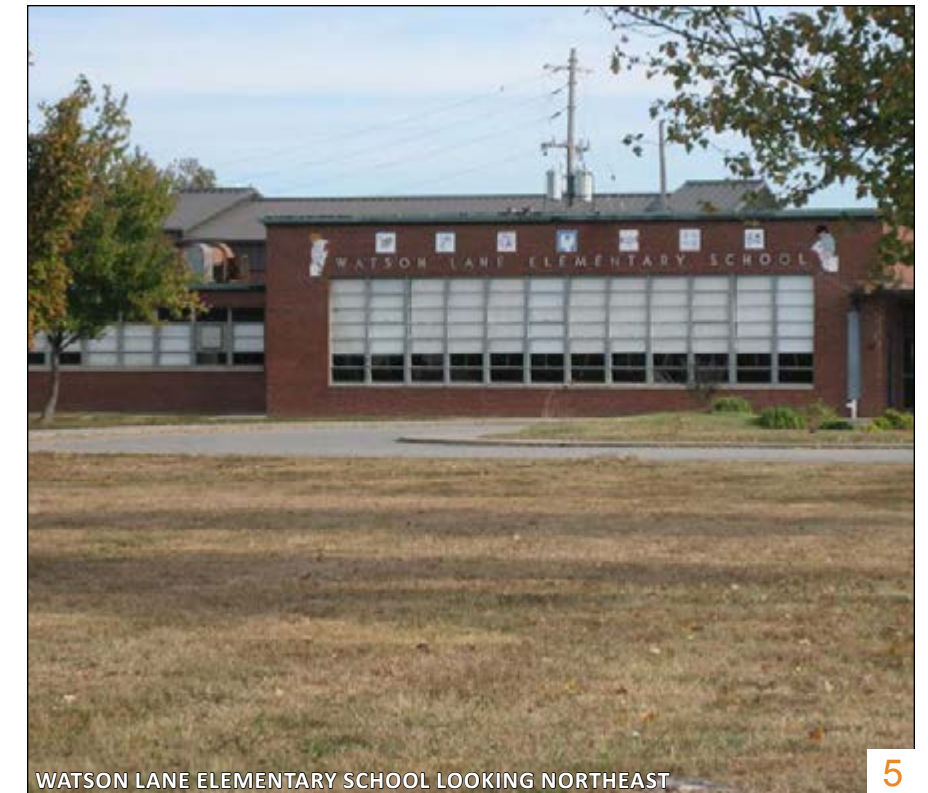
WATSON LANE ELEMENTARY SCHOOL LOOKING NORTHEAST
