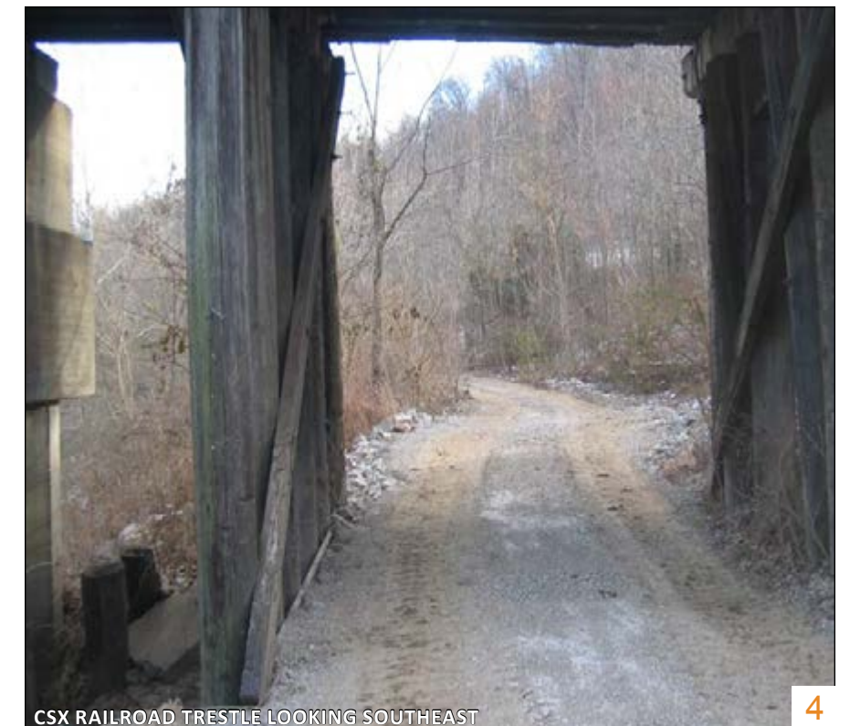
CSX RAILROAD TRESTLE LOOKING SOUTHEAST
