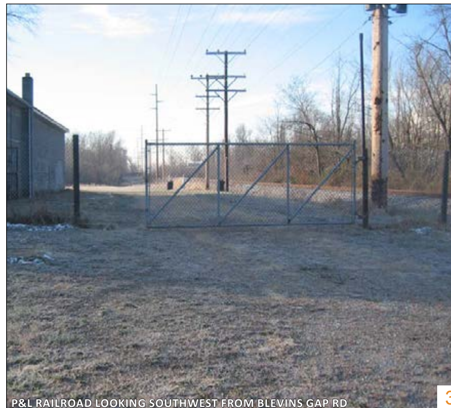
P&L RAILROAD LOOKING SOUTHWEST FROM BLEVINS GAP RD
