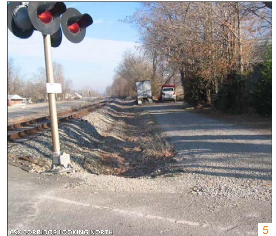
CSX CORRIDOR LOOKING NORTH
