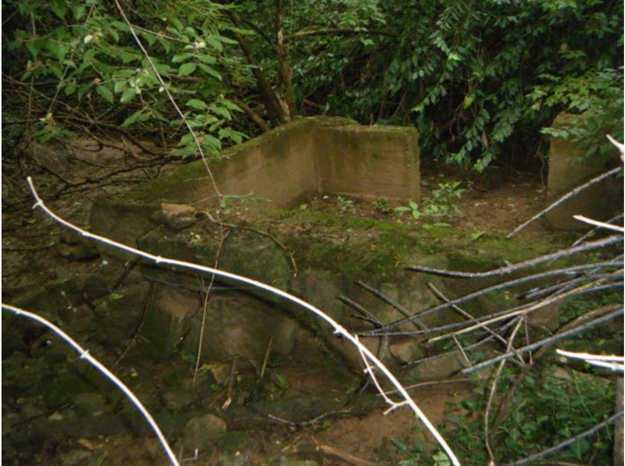
Figure 80. Limestone and concrete foundation at base of large sinkhole next to spring, facing west.
