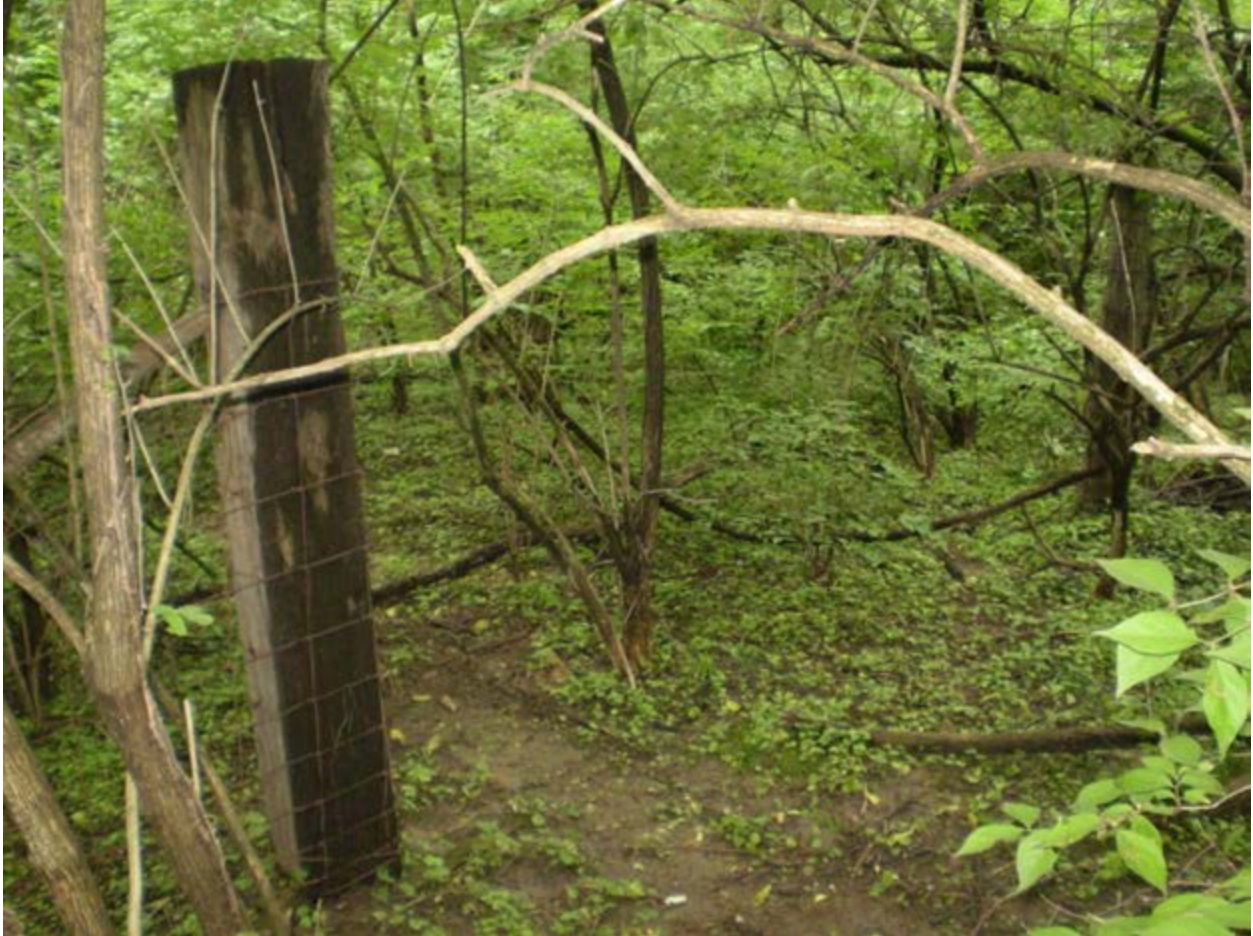
Figure 91. Old fence and fence opening enclosing concrete structural foundation, facing southwest.
