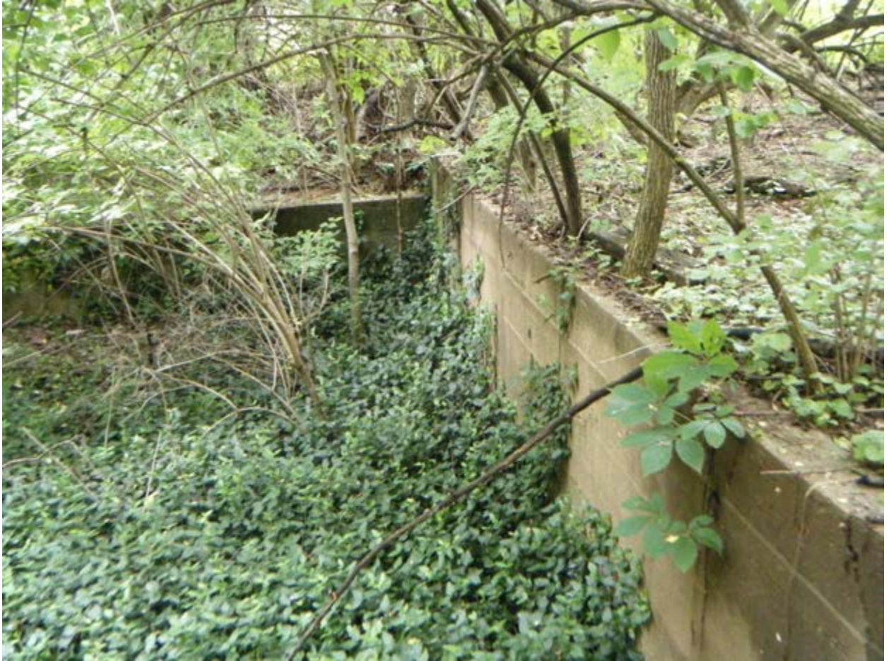
Figure 90. Structural foundation, facing west.
