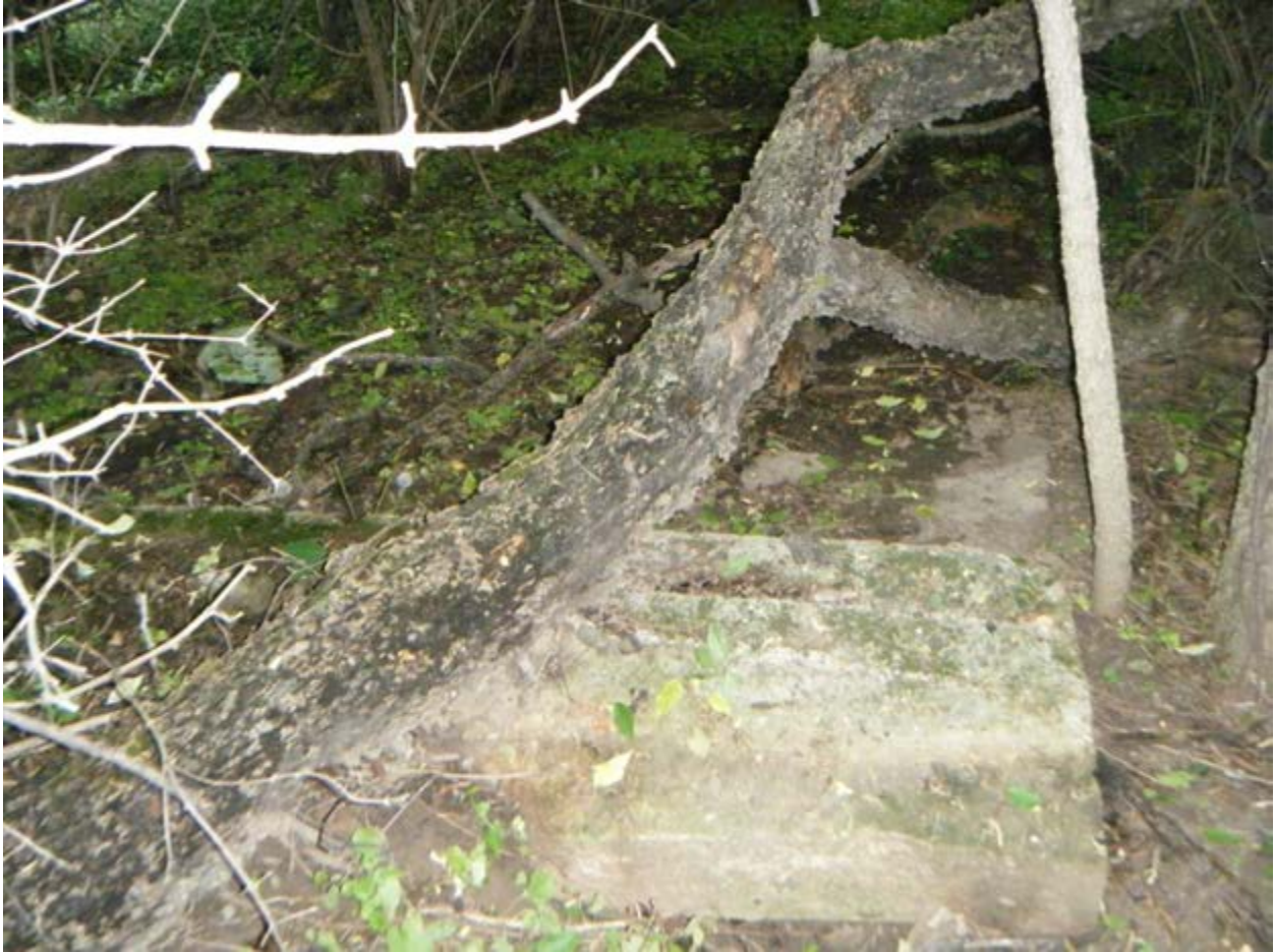
Figure 89. Poured concrete floor and foundation, facing east.
