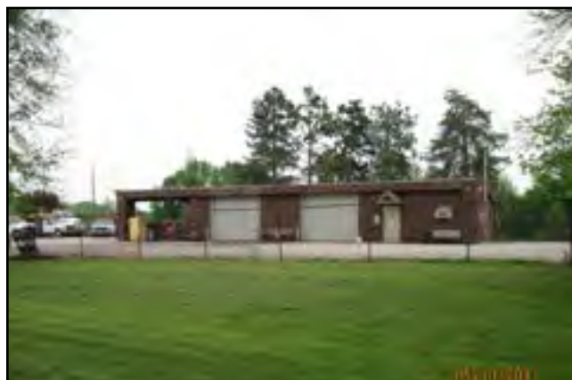
View of Metro Parks Maintenance facility from tennis courts
