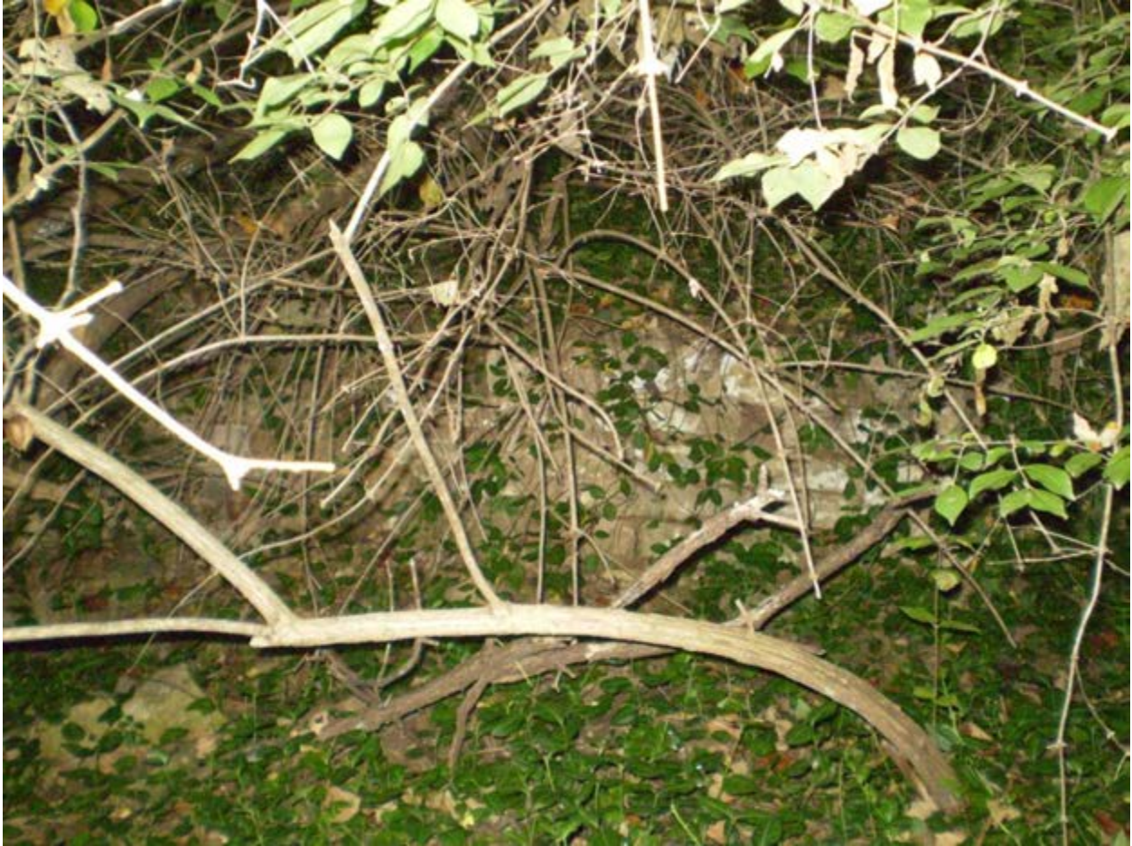
Figure 76. Southern foundation wall of house from within central depression, facing south.
