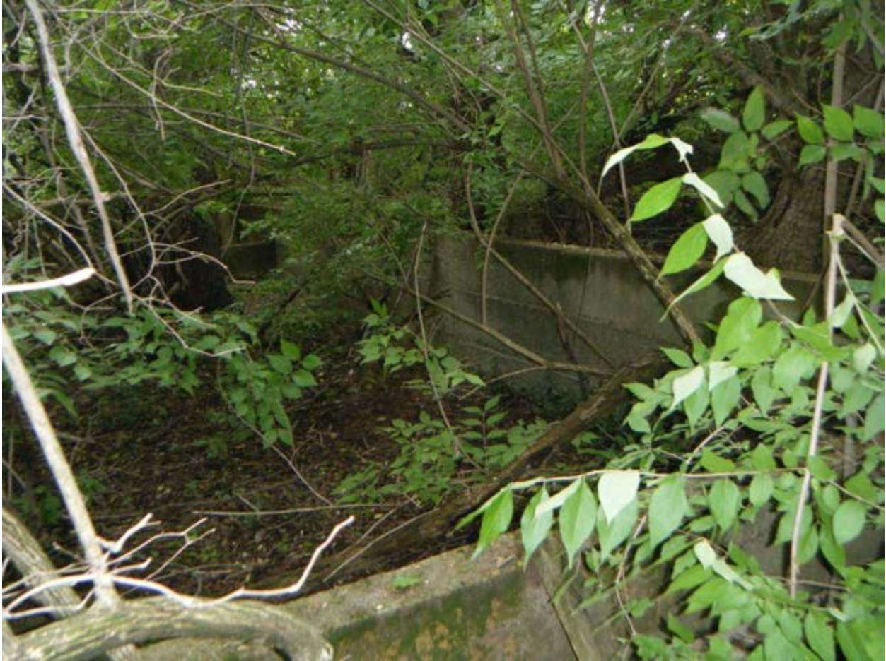
Figure 88. Concrete foundation of structure located in sloped and wooded area south of ball fields.
