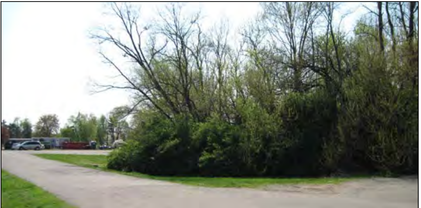
Major sinkhole located adjacent to main parking field
