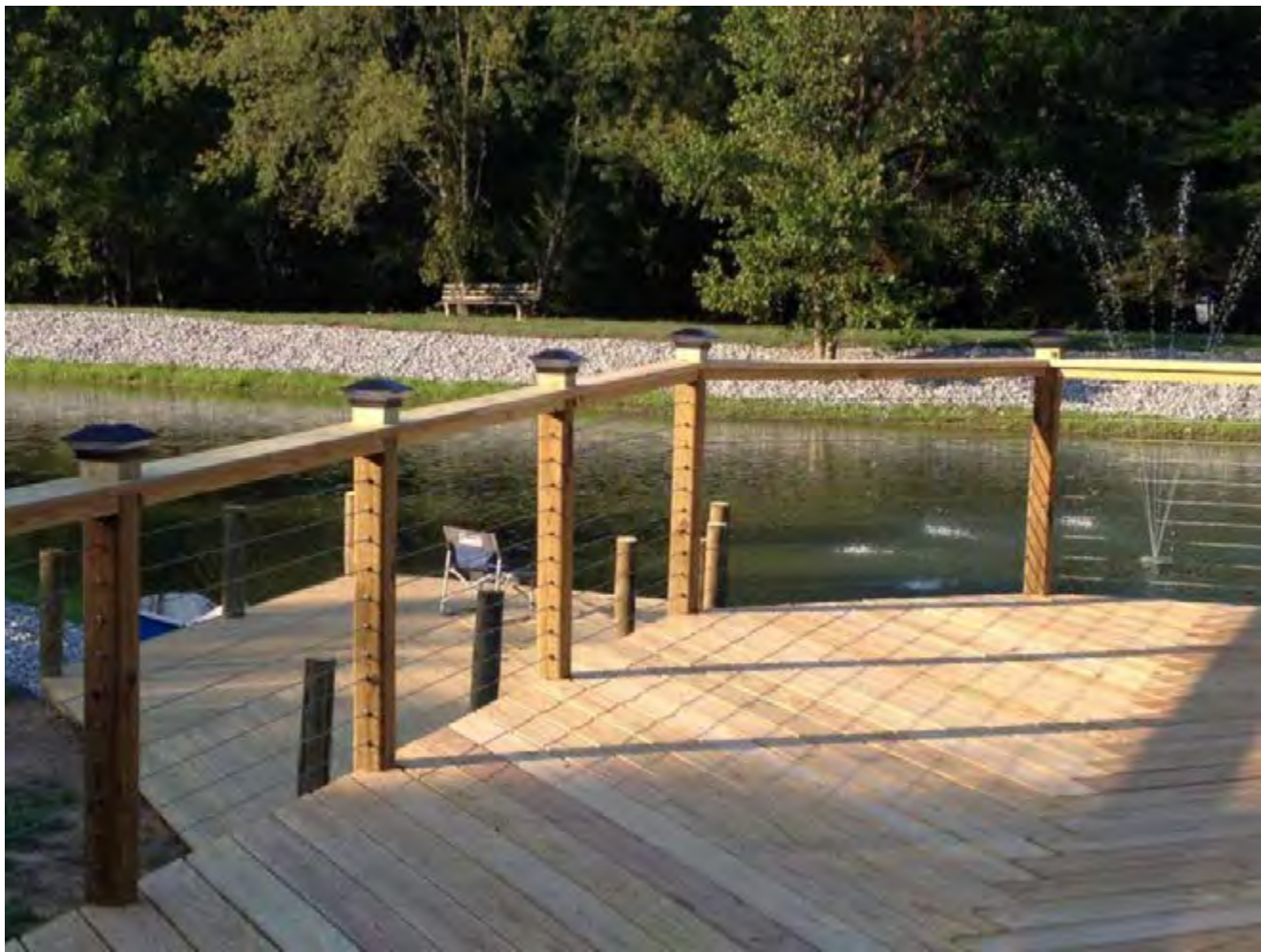
Lakeside Dock Area
